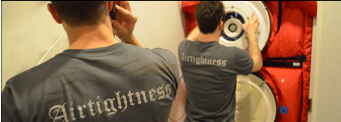
Blower door test preparation.
